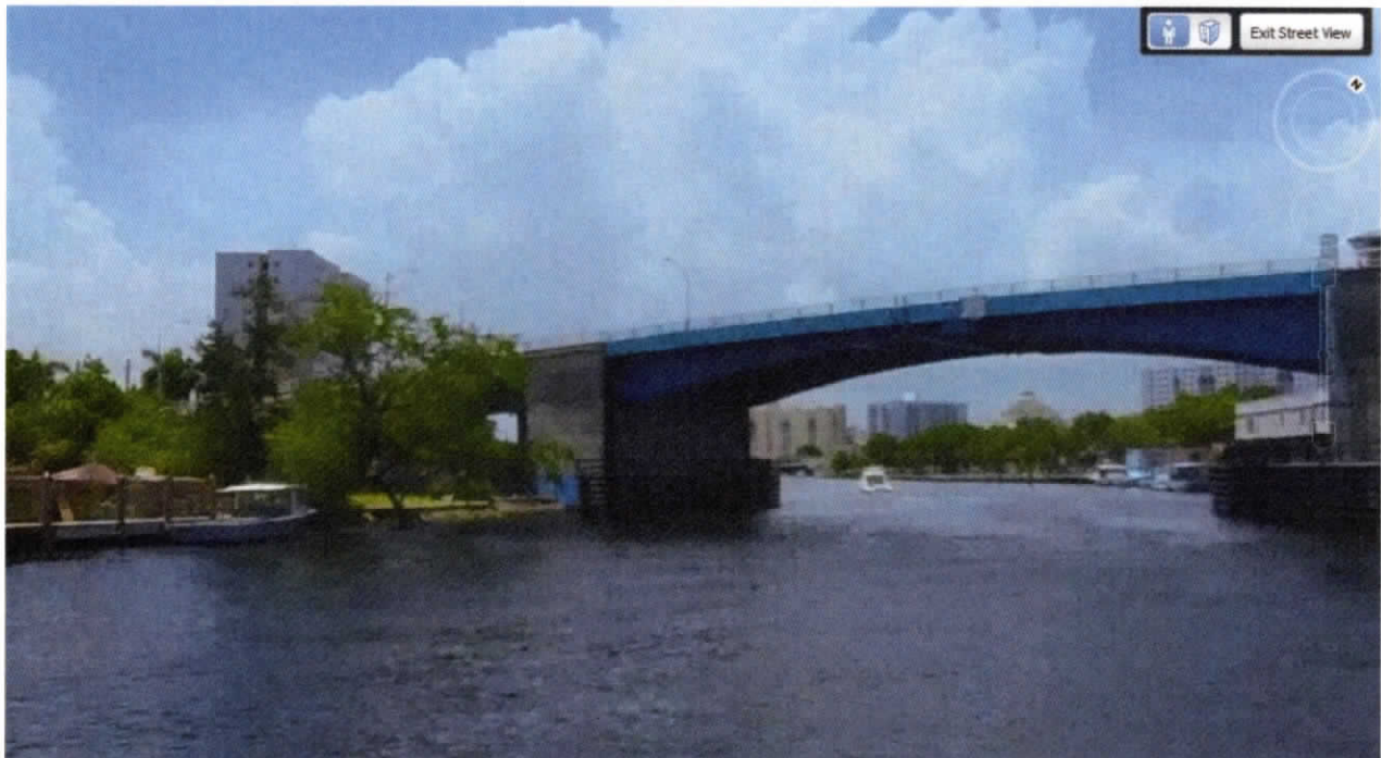
Flagler Bridge and New Park Area
